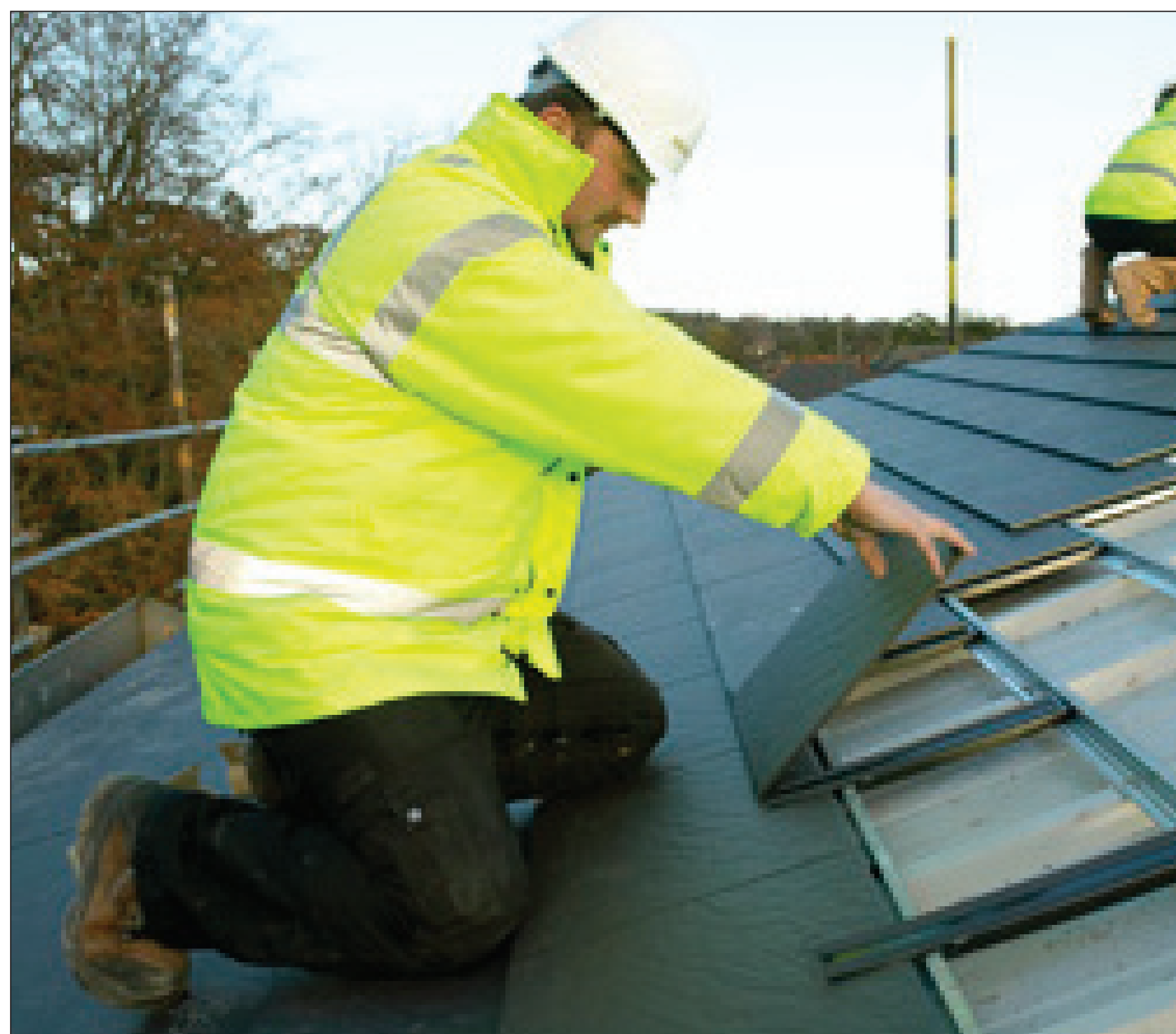
Nu-Lok's™ exclusive Ceramic Slate roof tiles simply click into place
