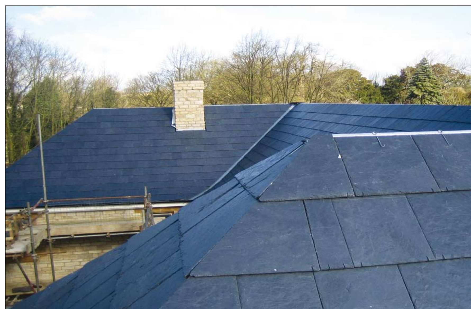
Nu-Lok TM slate created neat, sharp mitred hips
