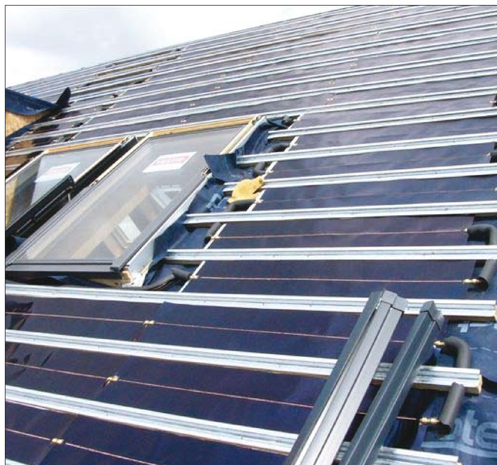
Green Frog TM solar hot water panels during installation
